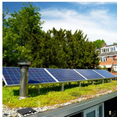
Figure 9: PV installations on the roof reduce heat gains of the building while supplying renewable energy
