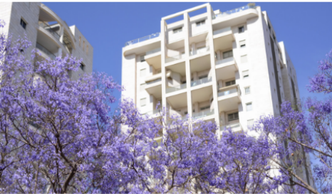
Figure 5: Light colours used on exterior building walls reflects incoming sunlight
