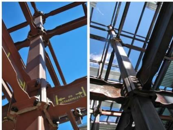
Figure 2.13. The ConX® System (Cradle to Cradle Certified Products Registry, 2014)
