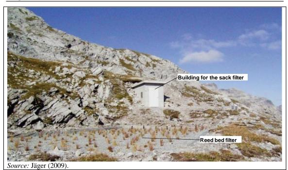
Figure 6.25: Example for a reed bed filter for the treatment of grey water from a hut at 2 245 m above sea level, designed for 30 PE60
