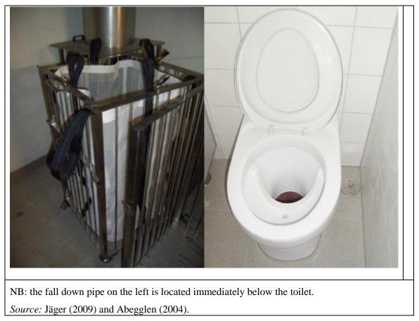
Figure 6.24: Separation toilet (on the left) and separate dry collection of faeces (on the right)
